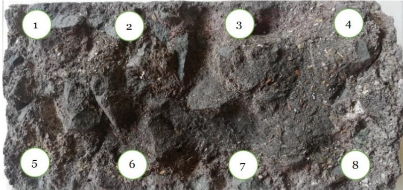
Figure 2. Sections in the fractured concrete where penetration depth of sodium chloride was measured.
